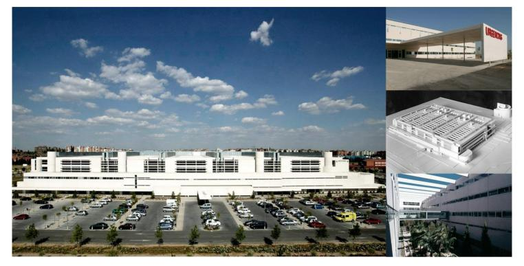
The Fuenlabrada Hospital has a surface area of 159.50 x 12300m on plan. From the beginning of the project, a pre-cast structure with rigid nodes and no expansion joints was considered.
